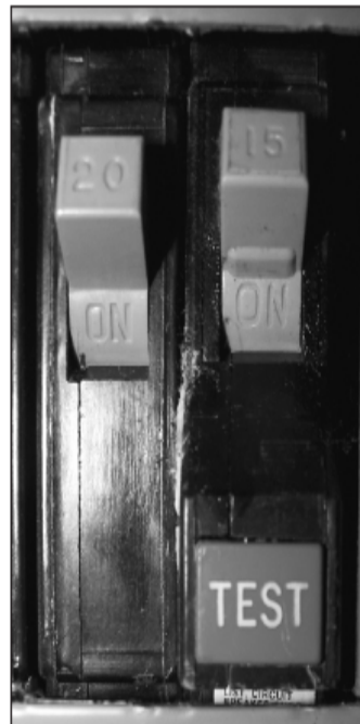
Ground Fault Circuit Interrupter (GFCI) circuit breaker
